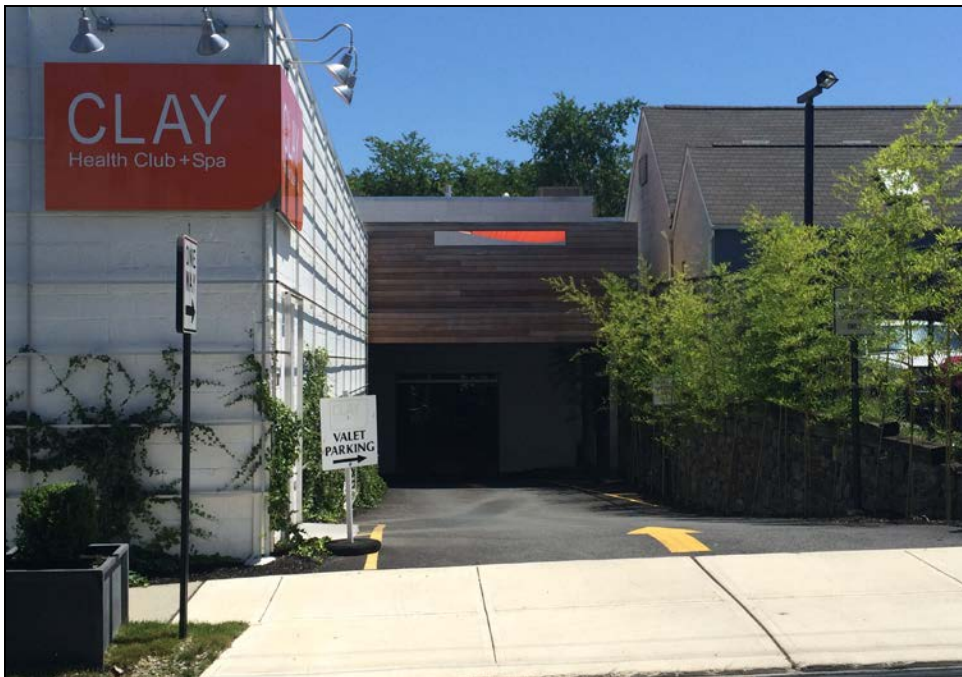
View of Entrance to Parking Garage
